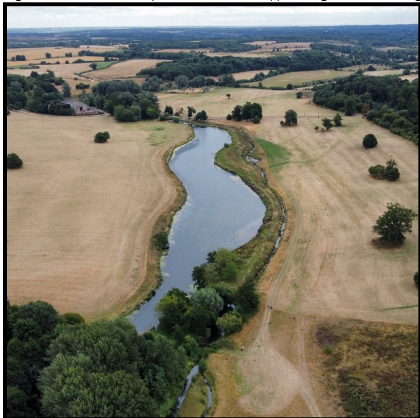
Figure 16. Aerial image of the Broadwater and the new adjacent bypass channel.
