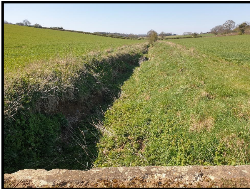
Figure 21. Dane End Tributary. Dry, straightened and deepened channel.
